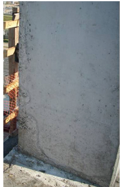
Results from a standard industry vibrator overspeeding
